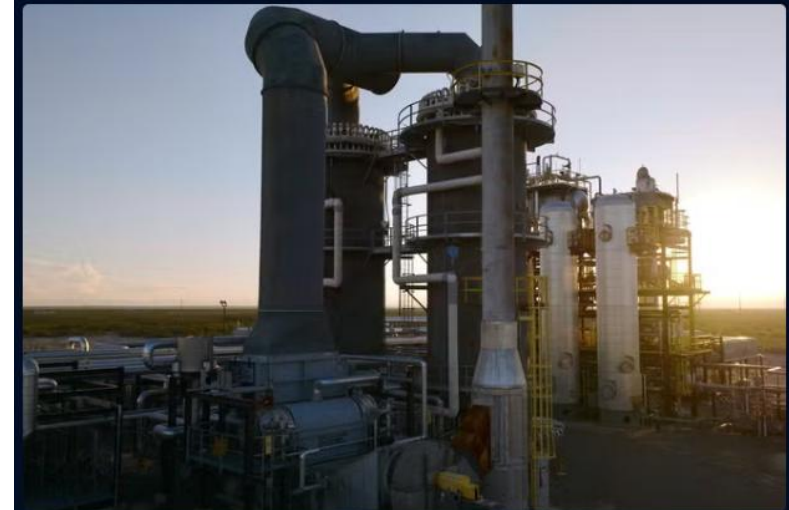
Project Roadrunner under construction in Pecos, Texas Photo: Infinium
